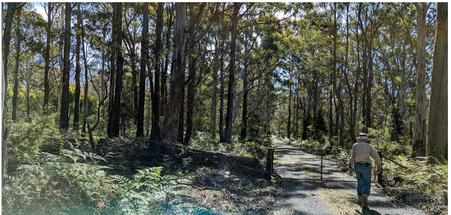
Good quality road infrastructure is an important risk management tool
